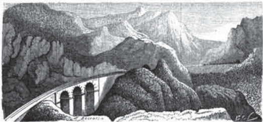
GRANDS TUNNELS DE GUADARRAMA.
